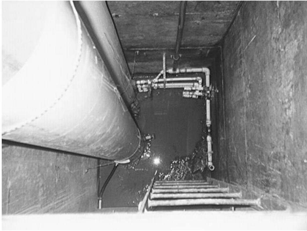
Note: the shelter for this type of installation requires a minimum floor area of  $7.5 \text{ m}^2$  (dry well floor area, assuming a  $0.31 \text{ m}$  diameter wet well, must be at least  $1.5 \times 2.0 \text{ m}$ ). The dry well must be fitted with a ladder bolted to the wall, a  $37.5 \text{ mm}$  floor drain and covered with a trap door or removable floor plates.
